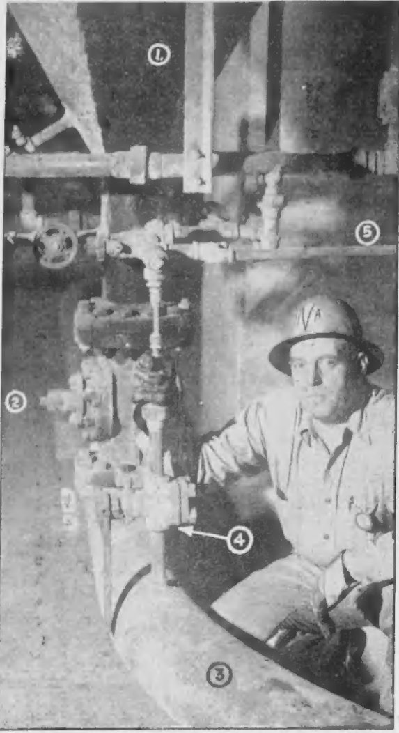
Top CYI Capital Award winner Hendrik van den Arend is shown at left with the suggestion that has earned him Fls. 1750, with an initial of Fls. 750 and the first capital of Fls. 1000. The idea: fresh catalyst must be transferred once a day from the Cat Plant hopper, No. 1, to the loading line, No. 3. Formerly the valve at No. 2 was used, loading through a six-inch line. Mr. van den Arend proposed loading through a small pipe (No. 4) with pressure from the air line, No. 5, with better control and less upset to the operation of the unit.
